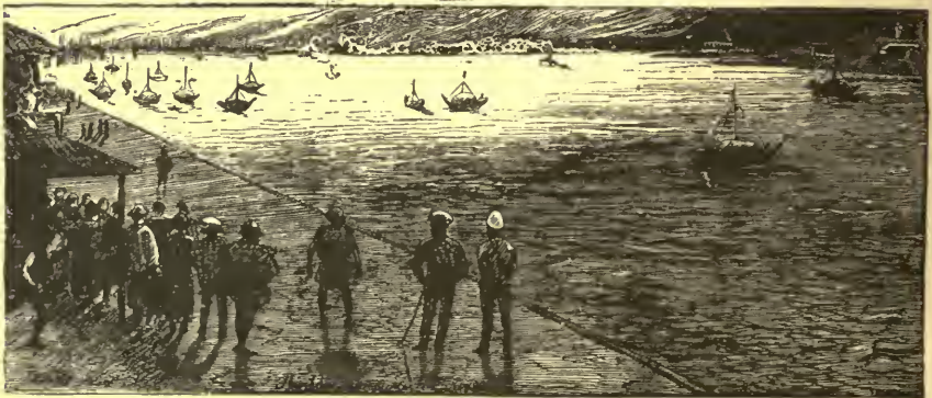
FIRE IN TOKIO, AS SEEN FROM THE BUND, YOKOHAMA.
